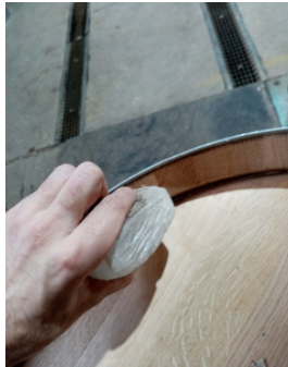
Melt the paraffin onto the leak.
